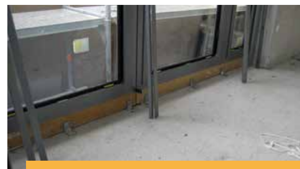
Phonotherm® 200 as highly resilient basic profile
