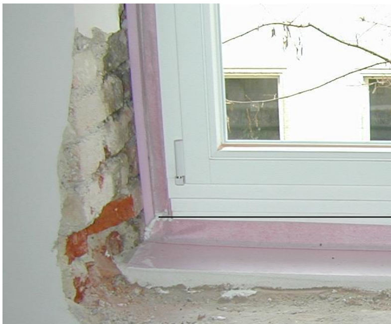
Fig. 7: Winflex® TFS or Winfix for sealing corners – tape ends are pressed firmly into the adhesive
