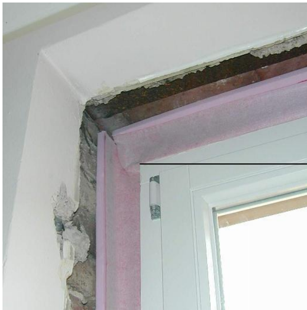
Fig. 7: Corner formation by applying Winflex® TFS or Winfix adhesive and for bonding the special adhesive strips
