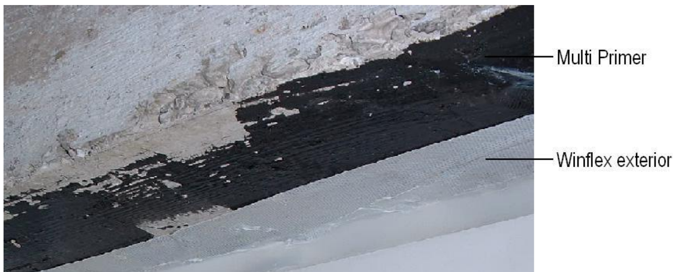
Fig. 3: reveal primed with Multi Primer
